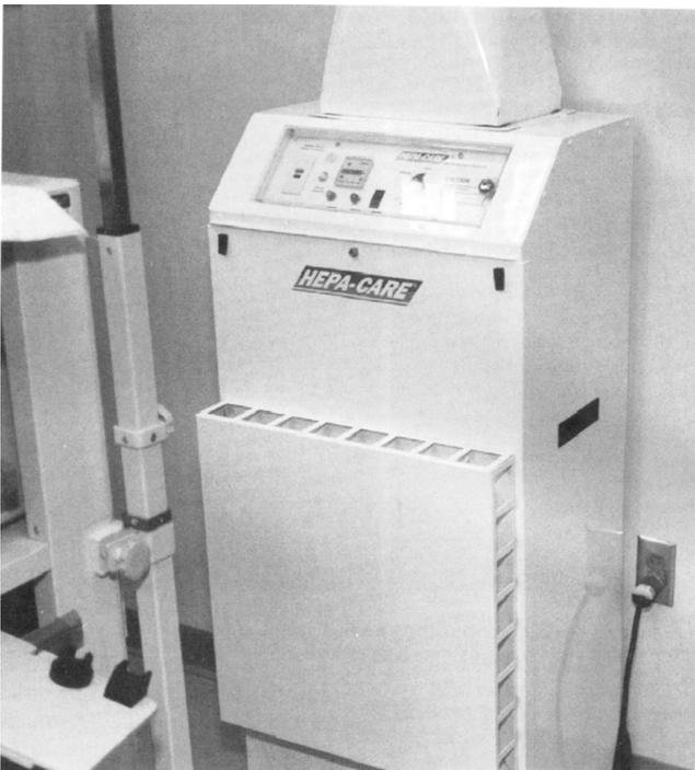
**FIGURE 3-6.** High-efficiency particle exchanger, such as the HEPA-Care (Abatement Technologies Inc, Atlanta, GA), which cycles room-volume air at least 14 times/hour.
