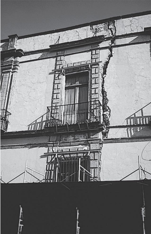
**Figure 6.11** The city of Mexico has subsided by many meters as a result of groundwater abstraction. Many of the ancient buildings in the city center have been severely damaged, and have been cracked and deformed.
