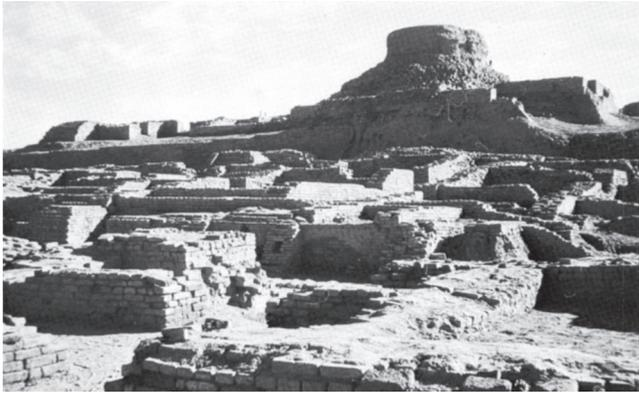
**Figure 6.14** The ancient city of Mohenjo-Daro in Pakistan was excavated in the 1920s. Irrigation has been introduced into the area, causing groundwater levels to be raised. This has brought salt into the bricks of the ancient city, producing severe disintegration.
