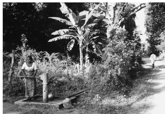
Fig. 1.8 Collection of water for domestic use from a hand-pumped tube well drilled in Precambrian metamorphic rock in the Uda Walawe Basin, Sri Lanka.
