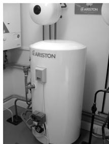
**Unvented system using expansion vessel**
