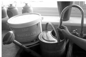
Hose connected to a tap without backflow protection (causing possible contamination)
