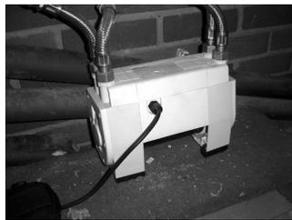
Flexible connections to reduce noise from booster pump
