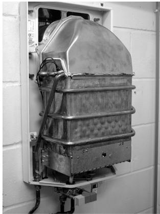
Multi-point heater with the case removed
