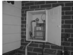
Typical Meter Box Installations
