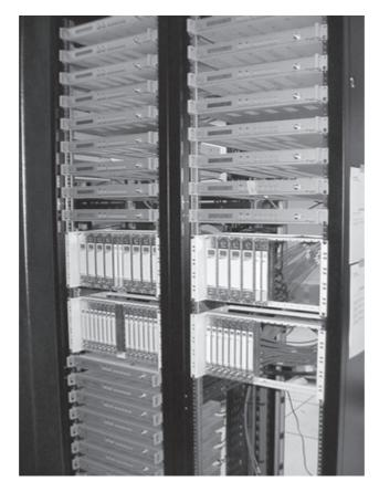
**Figure 1.2** Photo of headend-inside. Although headend buildings are seldom elaborate on the outside, inside they contain an array of sophisticated processing and transmitting equipment. [Photo courtesy of ATX]
