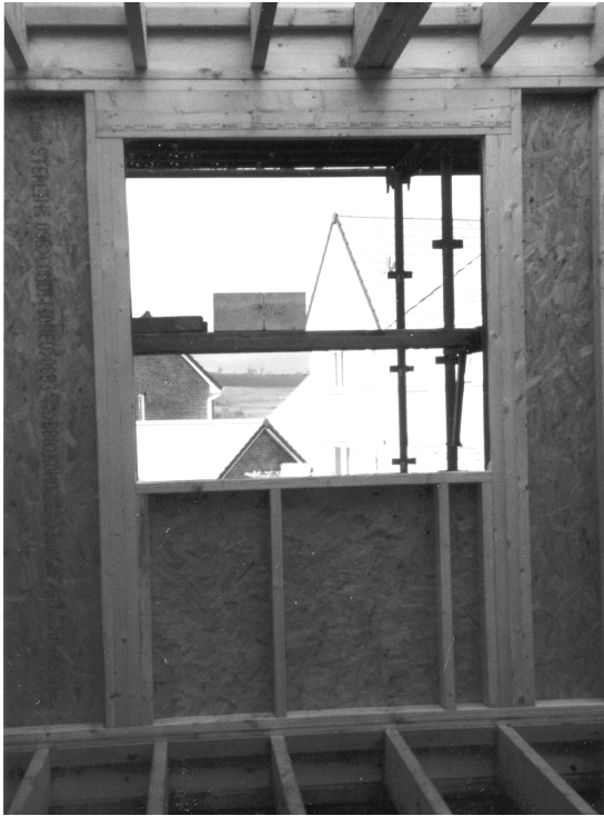
Fig. 5.41 Modern timber panel at window opening.
