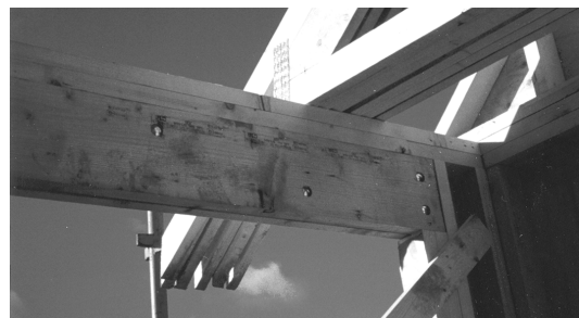
Fig. 5.44 Flitched beam over large opening.
