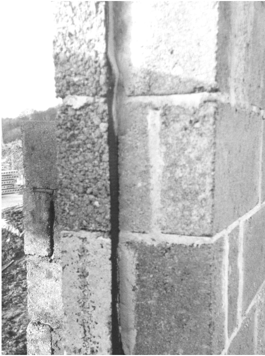
Fig. 5.11 Detail of checked jamb.
