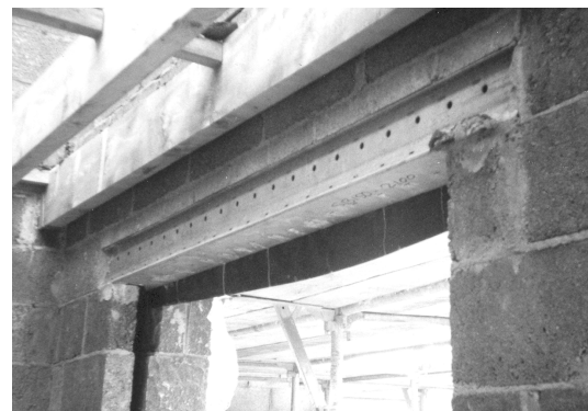
Fig. 5.10 Steel lintel at inner leaf of opening.
