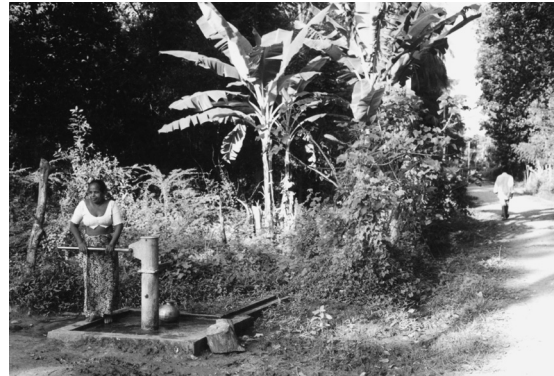
Fig. 1.8 Collection of water for domestic use from a hand-pumped tube well drilled in Precambrian metamorphic rock in the Uda Walawe Basin, Sri Lanka.
