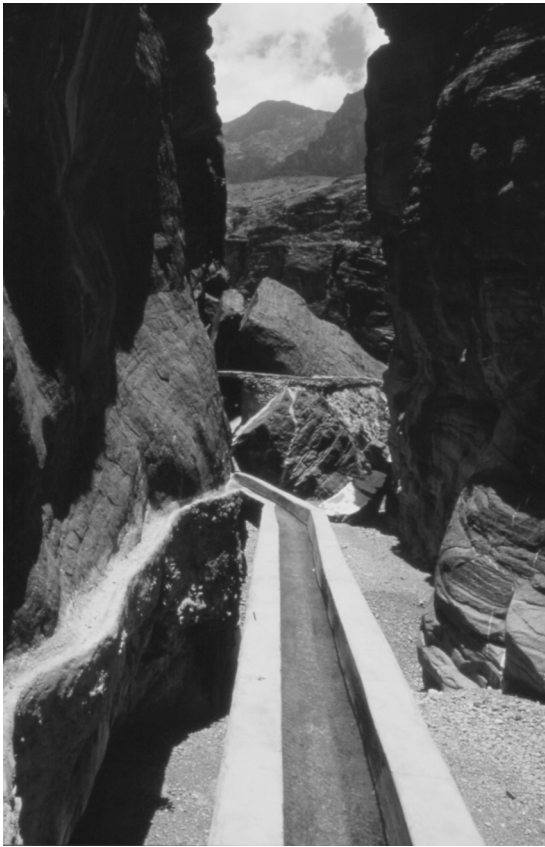
Fig. 1.4 Irrigation canal supplied with water by a qanat or falaj in Oman. Photograph provided courtesy of M.R. Leeder.
