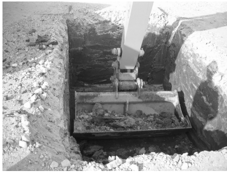
A The foundation is marked out and excavated to the correct level. The machine operator attempts to keep the sides of the excavation as true and square as possible.
