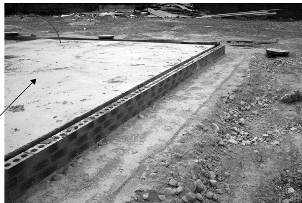
Photograph 3.2 Trenches and ground beams. Source: www.leedsmet.ac.uk/teaching/vsite
