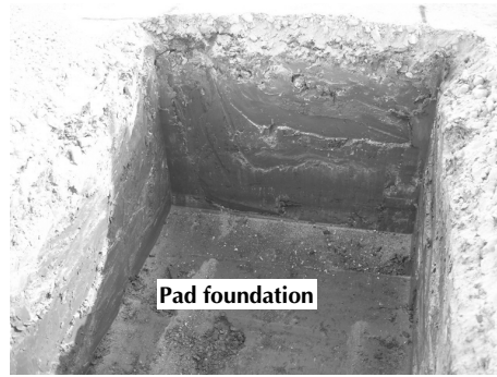
B This pad foundation has been excavated down to good loadbearing strata. The bottom of the foundation is clean and ready for inspection by the building control officer.
