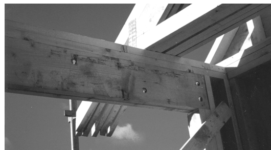
Fig. 5.44 Flitched beam over large opening.
