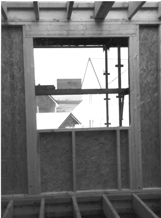
Fig. 5.41 Modern timber panel at window opening.
