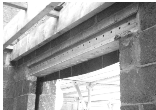
Fig. 5.10 Steel lintel at inner leaf of opening.
