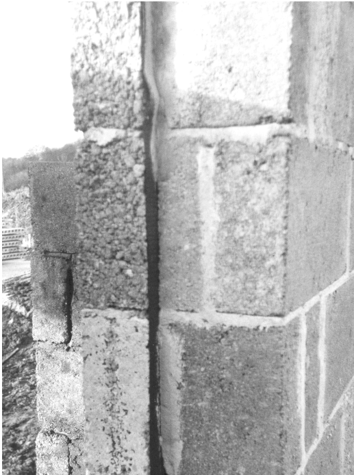
Fig. 5.11 Detail of checked jamb.
